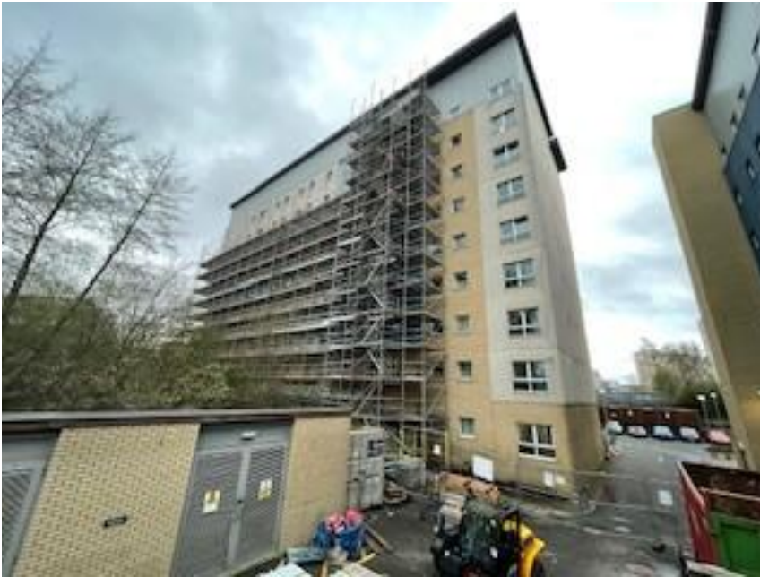
Phase 4 scaffolding ongoing
